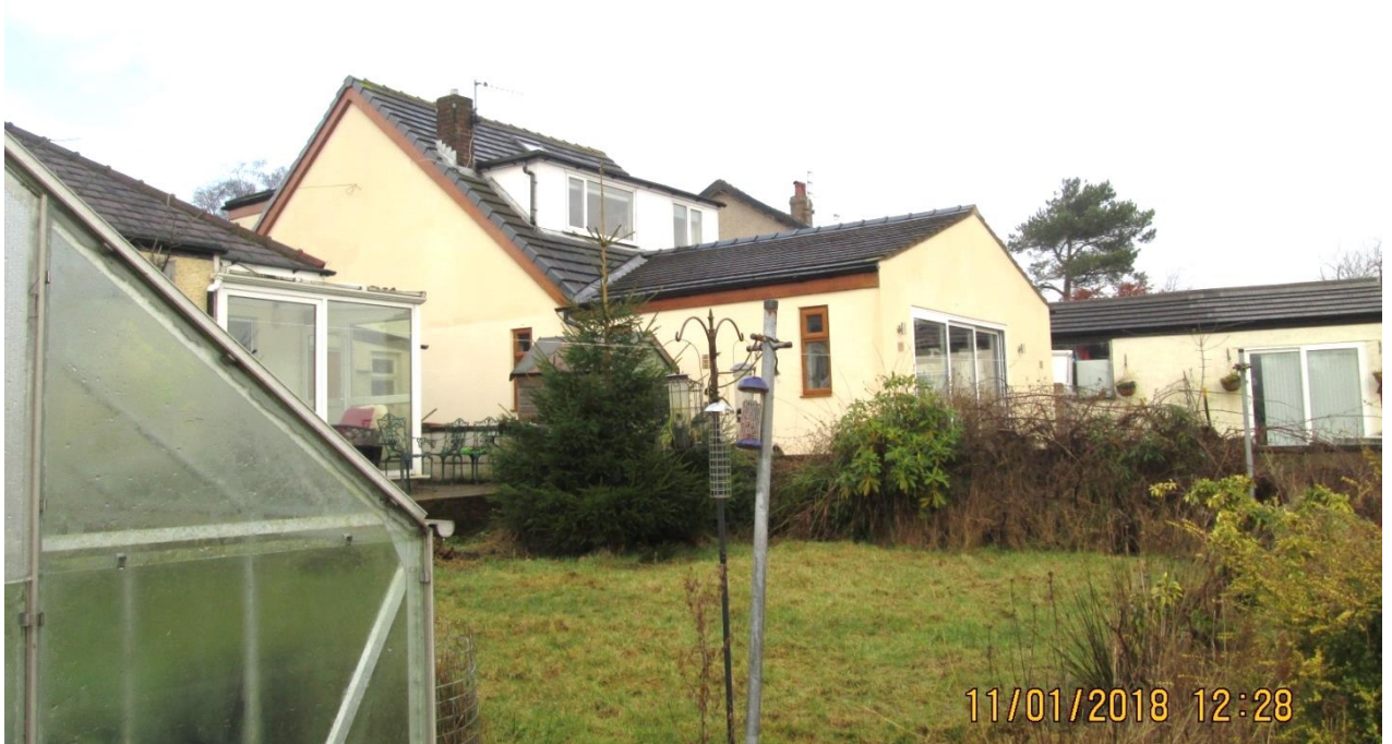
looking from the rear of the property towards no.70 Rosehill Road
